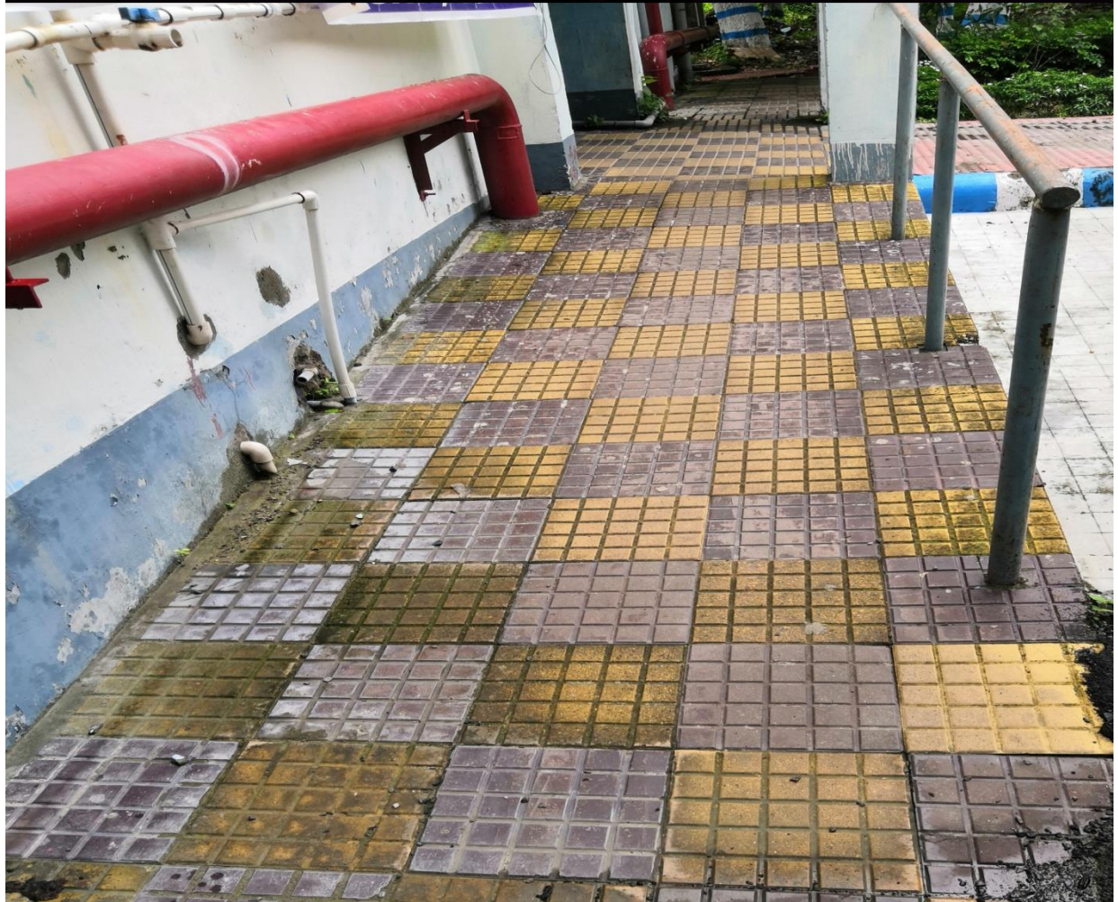
Ramp for easy access to classrooms
