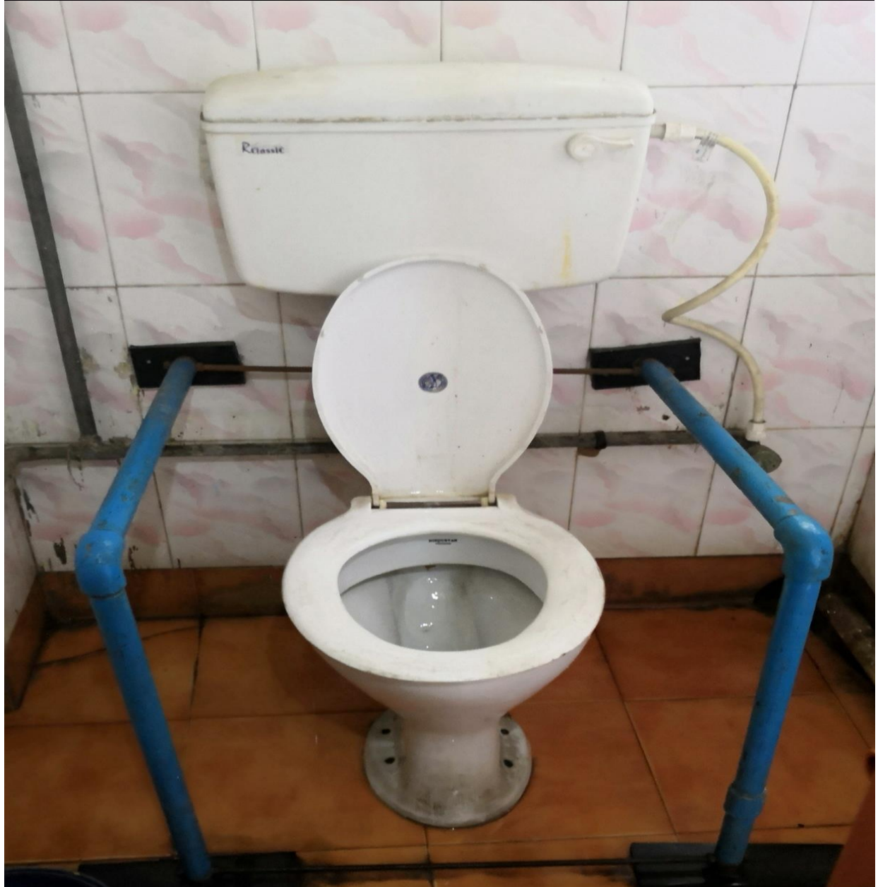
Disabled friendly Wash Room
